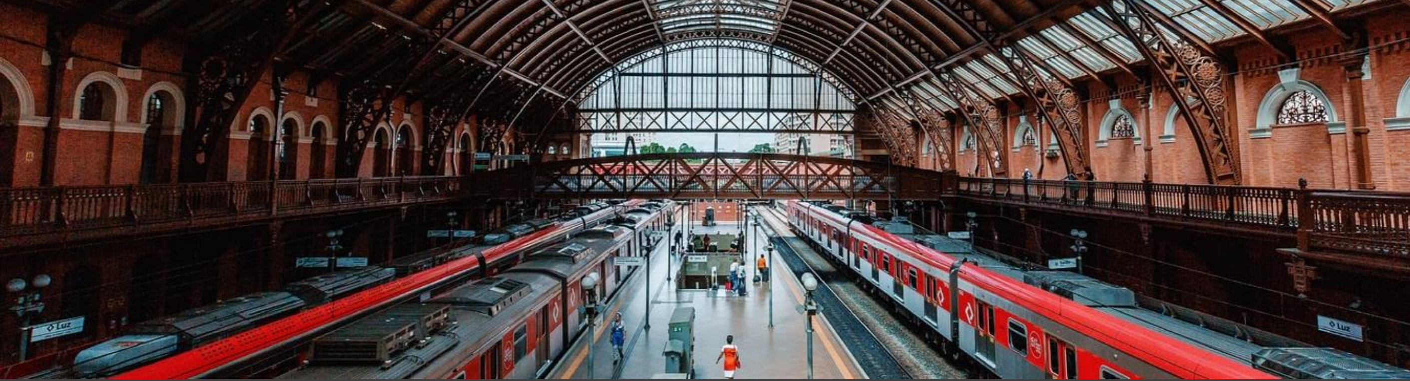
Luz Train Station, City of São Paulo
